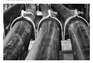
When installing SECON-X® Pipe in a trench, make sure that the pipe is at sufficient depth to protect it from surface traffic or other loads. At a minimum a layer of sand or pea gravel of 4 inch below the pipe and 6 inch above the pipe should be maintained.
