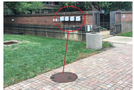
Unit can be mounted externally (remote monitoring)
