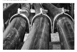
When installing FLEXWELL®-HL Pipe in a trench, make sure that the pipe is at sufficient depth to protect it from surface traffic or other loads. At a minimum a layer of sand or pea gravel of 4 inch below the pipe and 6 inch above the pipe should be maintained.
