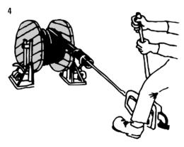
For large diameters or longer pipes, it may be necessary to use a simple hand-jack. If necessary, a deflection pulley can also be used. If you are using a motorized jack or tractor, ensure that the pulling speed does not exceed 1 ft/s.
